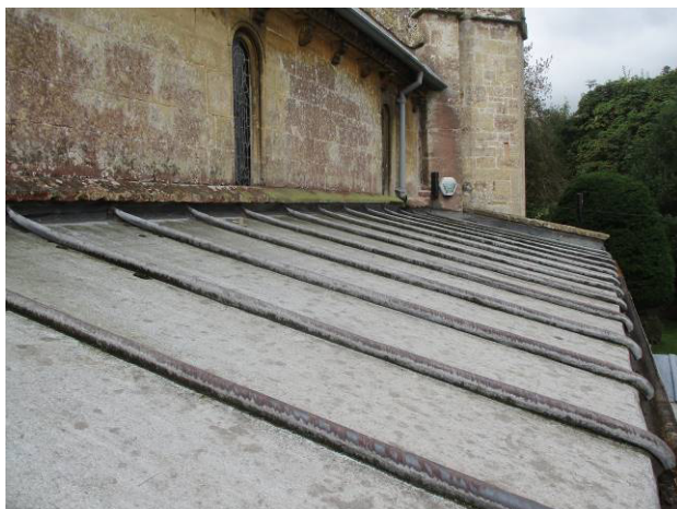
Fig.11 North aisle roof.
