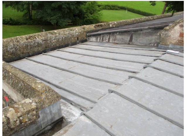
Fig.10 Organ chamber roof.
