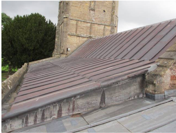
Fig.7 South aisle & nave roof.
