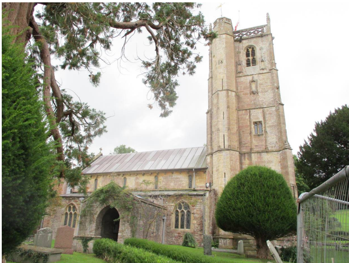
Fig.1 View from the north showing the tower, nave, north aisle and porch.
